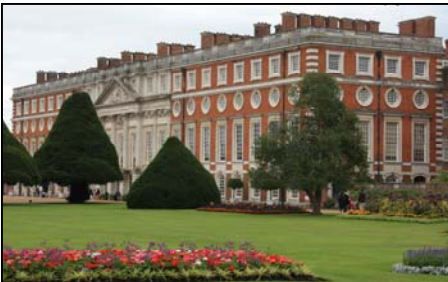
The South Façade of Hampton Court Palace
